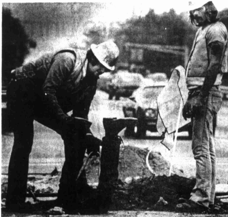
IN OVER HIS HEAD —The legs of construction worker Steve Gierny, center, of New Bedford, Mass., are all that's visible of him as he takes the head-first approach to repairing an excavated gas main in North Dartmouth, Mass. Lending a hand are Bob Conklin, left, of Fairhaven, Mass. and Bill Doberck of New Bedford.
