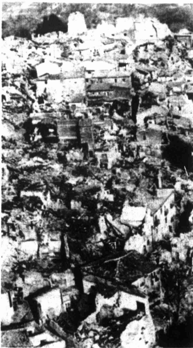
QUAKE DAMAGE — Airview shows the devastation caused by an earthquake that struck southern Italy Sunday leaving the town of San Mango Sul Calore nearly destroyed Tuesday.
