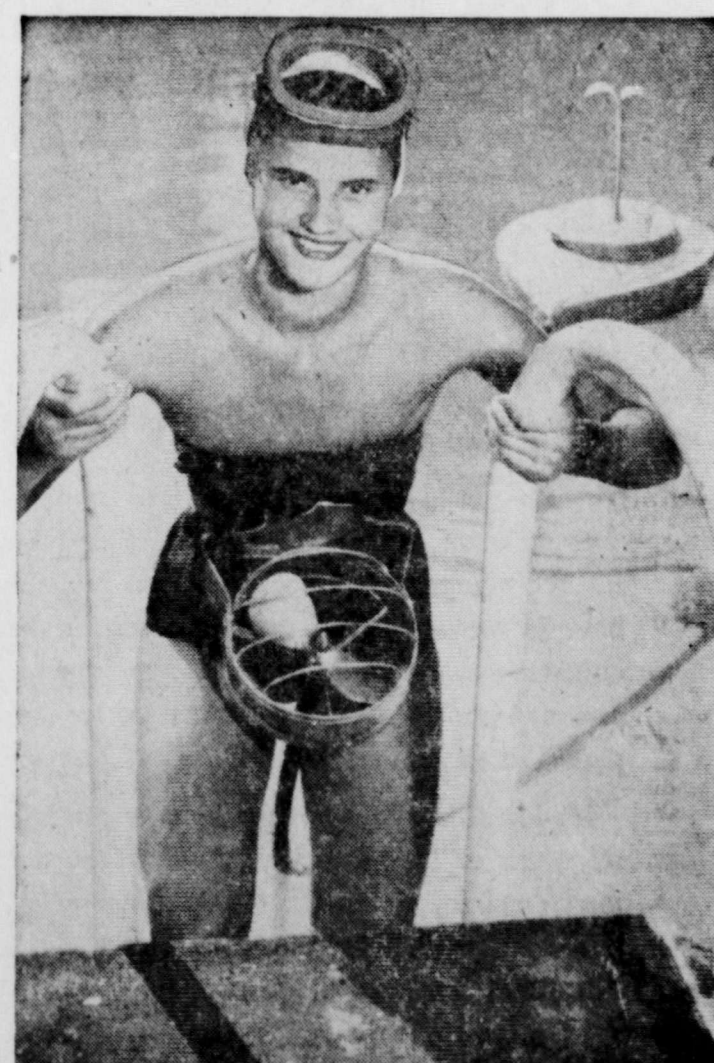
STROKELESS SWIMMER —A girl in Munich, Germany, exhibits a new gadget which enables her to swim 12 knots per hour without making a stroke. A 13-horsepower engine, housed in a boat-like dinghy (background), drives a small propeller tied to the swimmer's front by a cable and also pulls along the dinghy.
