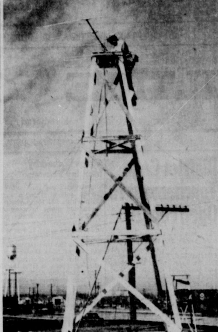
NEW AERIAL—Gus Henshaw, one of the first to try television in Perryton, is shown installing a new aerial on top of the Anderson Service Station on Brillhart, where he works. Gus says he gets programs about 50 per cent of the time, with the aid of boosters on the aerial and on the set. Reception was really good during January and he spent New Year's Day looking at a program in Montgomery, Alabama. Gus is a radio expert and has been a short wave "ham" for years.
