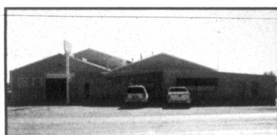
LARRY BAKER Plumbing, Heating & Air 11780 Hwy 152 665-4392
