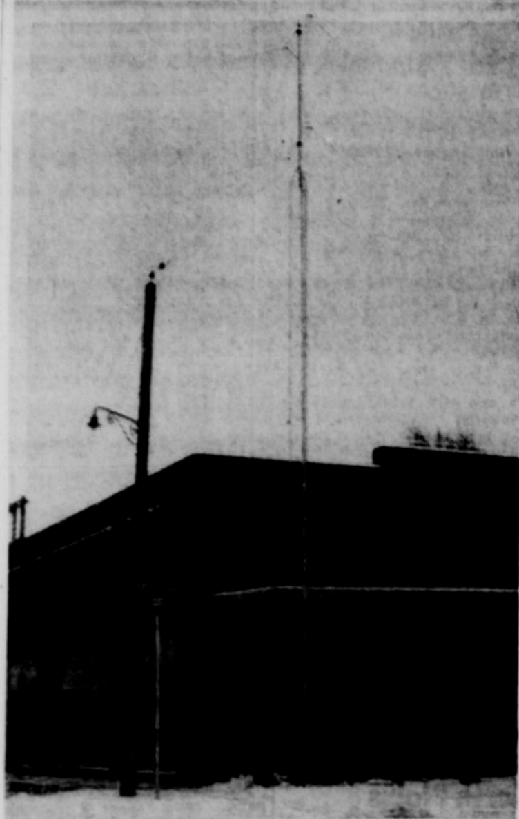
TELEVISION BOOM—Typical of the increased interest in television is this new metal antenna erected last week at the Good Furniture Co. by A. R. Macias. The Macias company is making the antennas at the former state highway warehouse south of Perryton and reports a booming demand for the new product.
