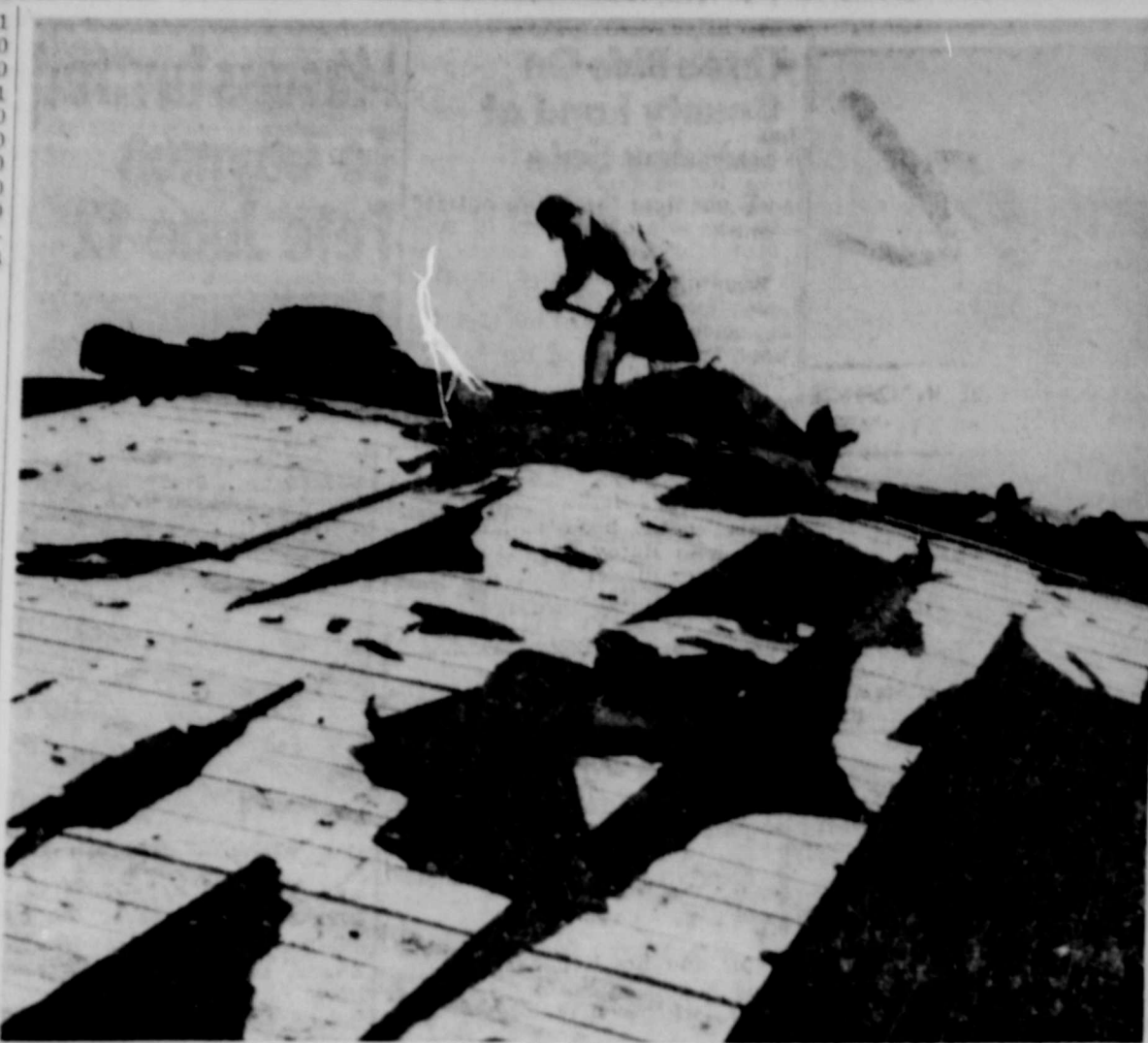
REPAIR ROOF—Earl Wurth, employee of Studevant Roofing Co. of Enid, is shown removing roofing paper from the roof of the Bethany school, damaged in the high wind Thursday afternoon. The storm followed a dust cloud that moved into the area at about 5 o'clock Thursday. Estimated damage, $1,800.
