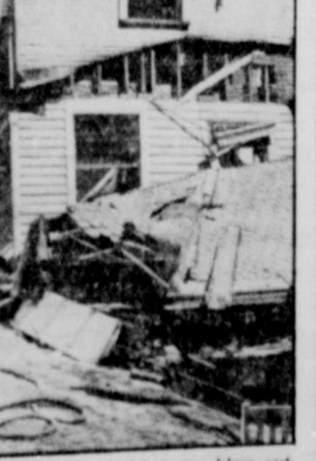
Explosion, believed to have been caused by leaking gas, blew out walls and buckled floors of this temporary frame school building at Barborton, O. More than 50 children were injured. Photo shows how blast shattered the structure. In foreground is one of many desks hurled through walls.
