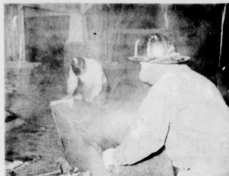
FIREMEN BATTLE BLAZE at 316 Hayworth Tuesday night. Considerable damage was reported.
