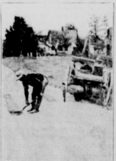
Patrolman Patching State Road.
