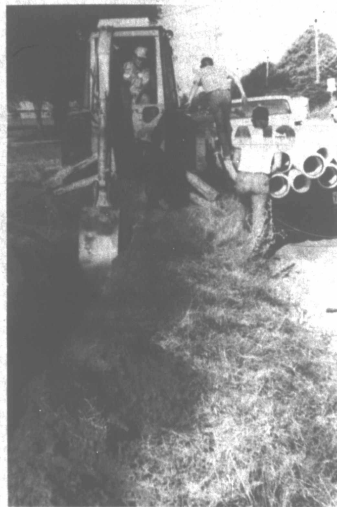
CITY CREWS were busy this week installing a new, larger water line on Sixth Street, west of Austin. The new line will provide better water service to residents in that area.
