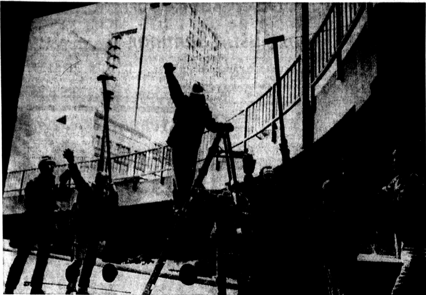
LIFTING, NOT WAVING — The photographer appears to be getting a friendly wave from a group of workmen at a new office building going up in Omaha. But the men are dead serious about handling a 600-pound piece of glass sched-
