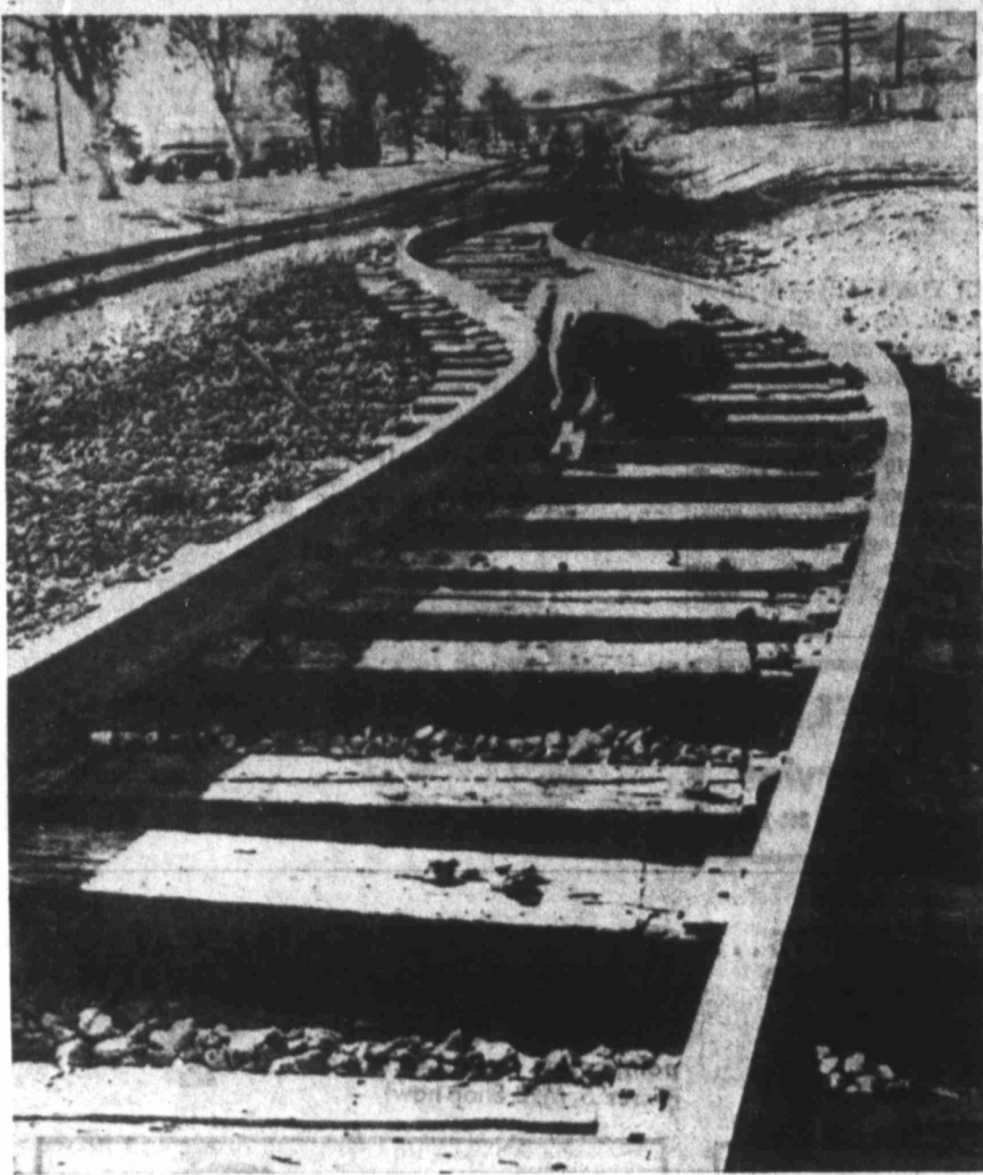
THE POWER OF A QUAKE — Twisted railroad tracks in front of the nearby San Fernando Valley Juvenile Hall give evidence of the force unleashed by the severe earthquake which hit Southern California Tuesday.
