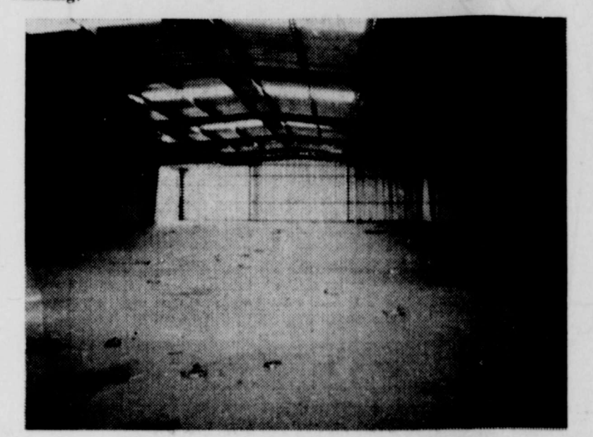
NEARING COMPLETION on Sixth Street at Avenue H is the City of Abernathy's new all-steel storage and shop building. Top photo shows the steel frame work of the 50x135-ft. building while it was being built. Photo below shows the interior of the structure with its concrete floor. The city will store its trucks and other rolling stock in the building when they are not in use. Also, a portion of the building will be used as a shop for water meter repairs and repairs on other city-owned equipment. Many of the items which clutter the north side of the city square will be moved to the new building.
