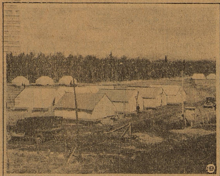
In Matanuska Valley, Alaska, future home of a small army of American colonists, a rugged, snow-capped mountain range is a silent witness of much hustle-bustle, as colonists, aided by transient workers, speed building of their homes before snow flies. Headquarters tents for the workers, located at nearby Palmer, are pictured above.
