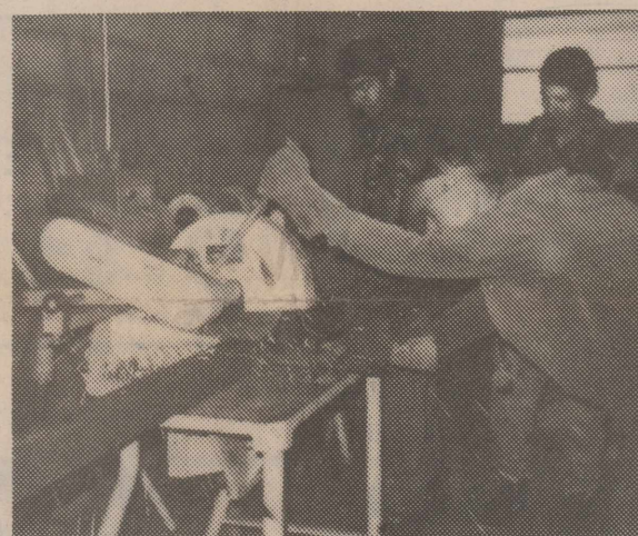
ROBY FFA: Cutting c-purlin for porch steps is Bobby Wilhite, Danny Castillo and Larry Castillo.
