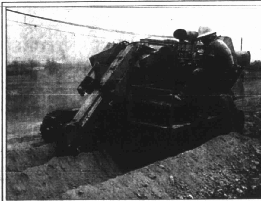
A heavy equipment operator runs this trencher to open a trench in which cable will be laid. The project is north of Big Spring alongside U.S. 87.
