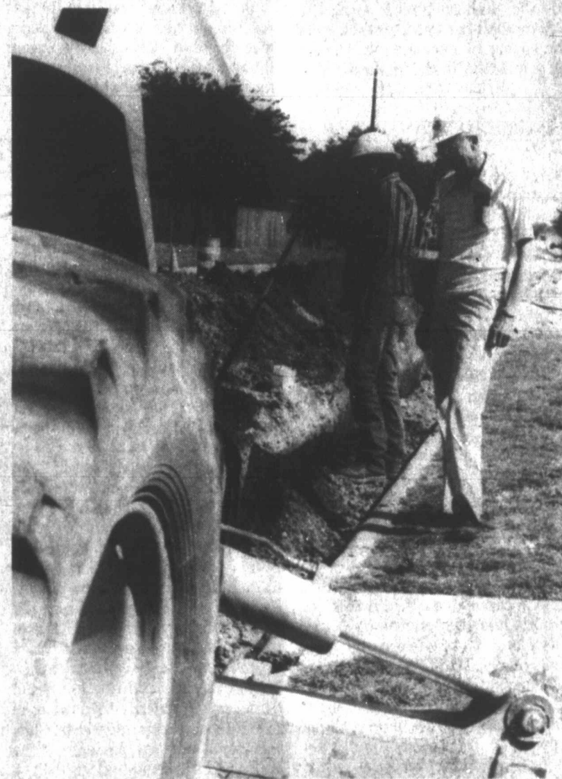
WATER LINE OBSERVER: Howard Taritt (right) looks over work on the waterline on Eastover St. Humberto Chavez of Rhode Const. mans the shovel on the work to replace a line that was frequently ruptured. City workers along 17th and that area had to follow the path of least resistance in installing the line and also route around other utilities rights-of-way.
