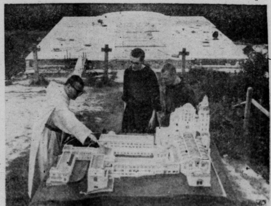
LOOK TO THE FUTURE —Benedictine monks discuss the details of a model of the new Prinknash Abbey they are building in western England. In background is the finished four base of the crypt. It will take more than a generation to complete the abbey.
