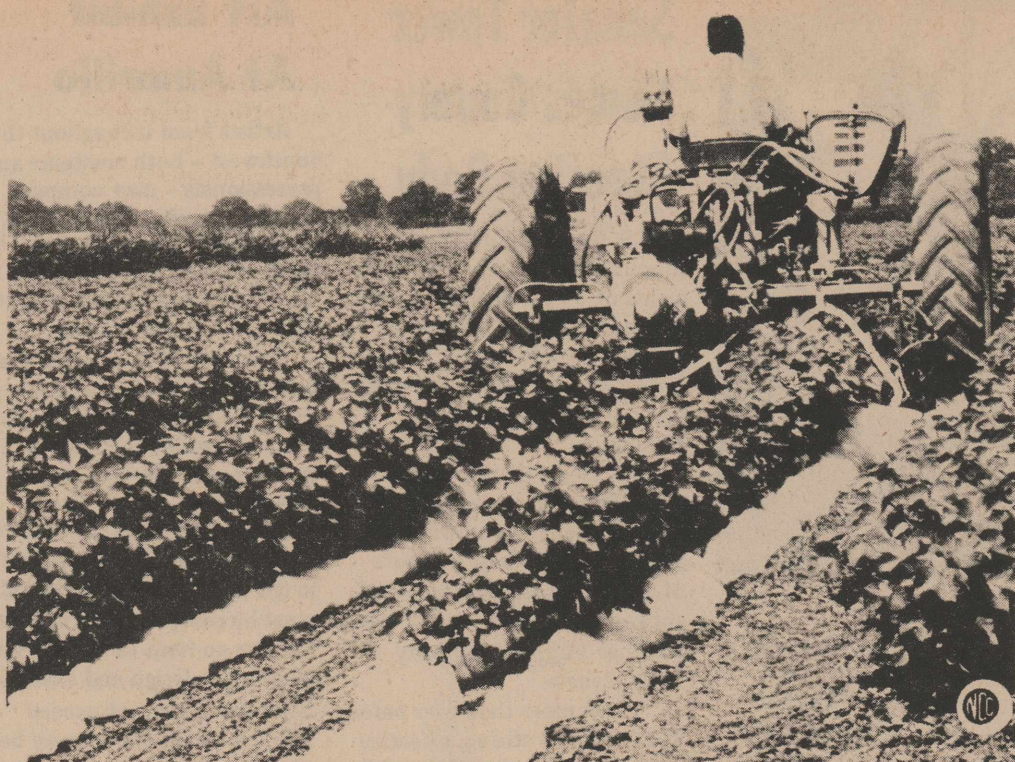
FOAM ON THE RANGE? —Herbicide-laden foam with the consistency of shaving cream makes a 'security blanket' around cotton plants in this field at the Mississippi Delta Experiment Station. The
