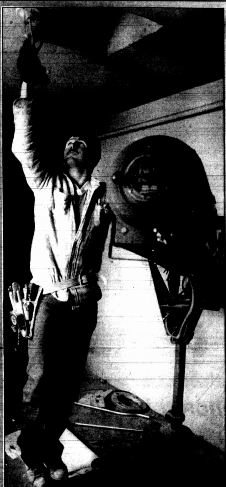
Tom Brown, of Brown & Associates electrical contractors of Big Spring, is seen as he reaches to remove a light fixture during renovation work at the Municipal Auditorium Tuesday morning. Electrical work in the Auditorium should be completed Friday, and acoustics work should begin this week, Public Works Director Tom Decell said this morning. Acoustics work includes painting, new floors and woodwork and trim restoration, he said. Construction renovations should be finished by the end of the month. Other improvements, including the possible addition of air conditioning, may be completed later. Decell said, work will not begin until work is complete, Decell said, explaining his reasoning about the use.
