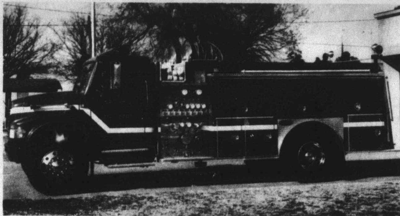
NEW FIRE TRUCK FOR TAHOKA FIRE DEPARTMENT - Due to the generous donations of many area citizens, through their $3 monthly volunteer donation on the city water bills, the Tahoka Volunteer Fire Department was able to make a sizeable down payment on this new fire truck for the department. Delivered recently to the city, the new $124,000 truck can pump 1200 gallons of water per minute, and firemen are currently training to familiarize themselves with the new equipment on the truck. The fire department continues to seek donations, however, to make payments on the new truck. (LCN PHOTO)
