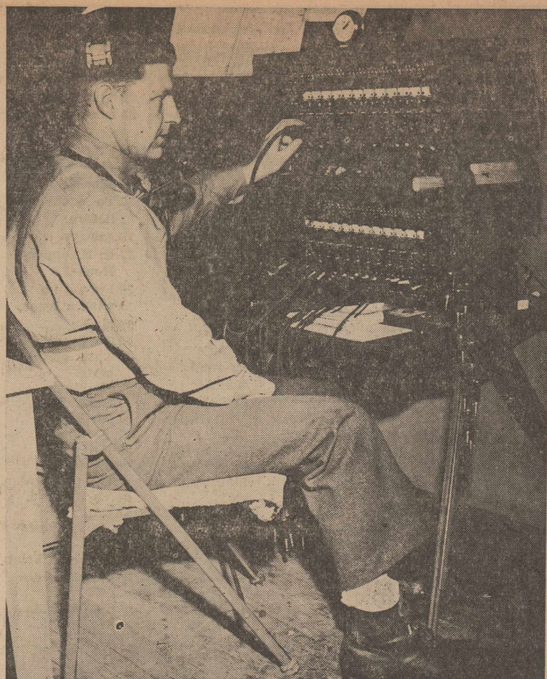
PRIVATE FIRST CLASS CLOISE E. DUNCAN Answers "Marine switchboard" to calls coming through here. Pfc. Duncan was a member of the Marine communications section at Dutch Harbor, Alaska, and operating the board is but one of the many tasks he has to perform. Cloise was home on furlough several weeks ago visiting his parents, Mr. and Mrs. H. L. Duncan. He is now stationed at Bremerton, Washington.
