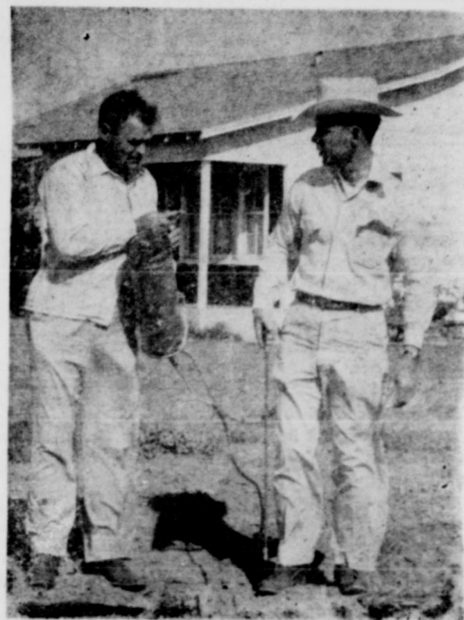
ONE-MAN SPRAY —Gerald Hanson, right, Martin County farm agent, demonstrates to Elma Nichols, Stanton farmer, one-man hand spray used for killing Johnson grass in cotton. Hanson designed spray which was made by Stanton machine shop. Hanson holds applicator stick, a metal tube, which is operated by a thumb valve. Naptha and diesel fuel mixture is used to kill the grass.
