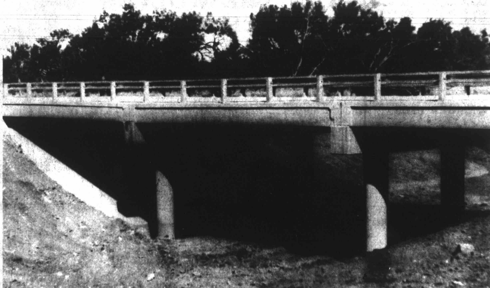
COMPLETED PROJECT - This is one of two recently completed bridges in precinct 2 that spans Morgan Creek. The bridges are located on county roads 290 and 280, three miles north of Iatan. Also under construction is a bridge spanning the Colorado River next
