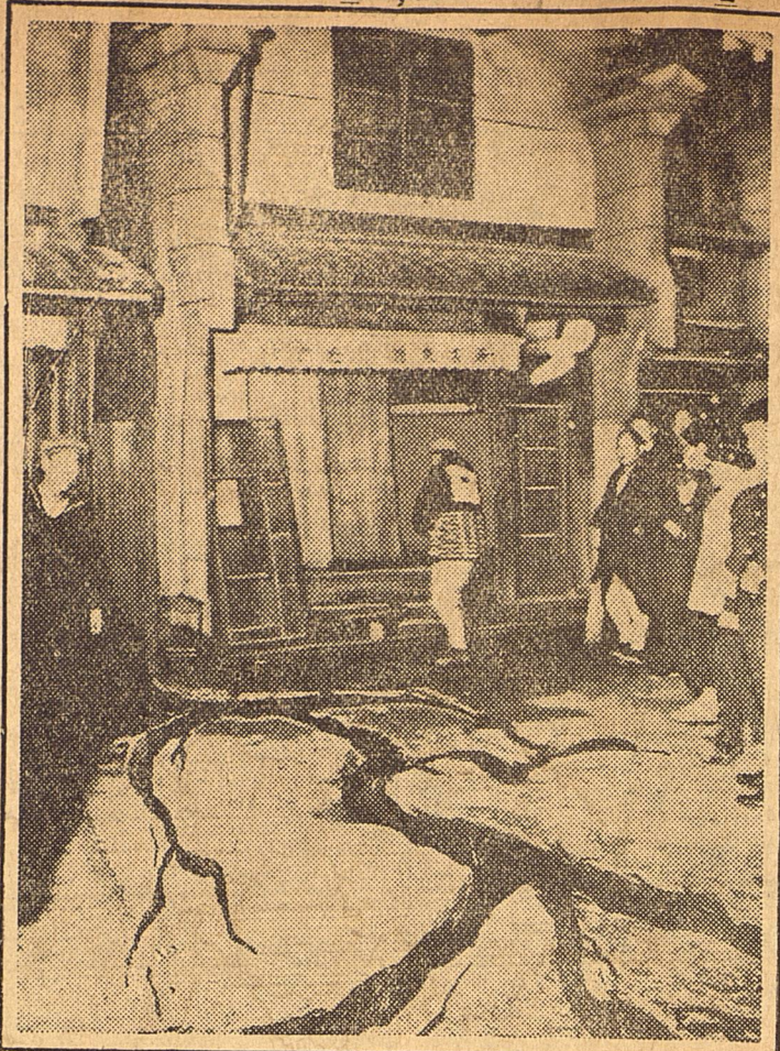
—NEA, Tokio Bureau A tremor which rocked the central part of Japan on March 7, de- molished several towns and claimed more than 2,000 lives. This pic- ture, taken at Osaka, shows the great cracks rent in the earth by the quake. It clearly shows how difficult it is to construct buildings that will withstand Japanese quakes.
