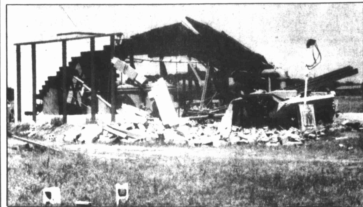
'Going, going . . . Stanton officials have been busy demolishing unsafe housing units around the city. In the top photo, a house located at the corner of West Broadway and North St. Charles is being demolished by David Thomas of Big Spring. The city's dog pound, bottom photo, also is being demolished.
