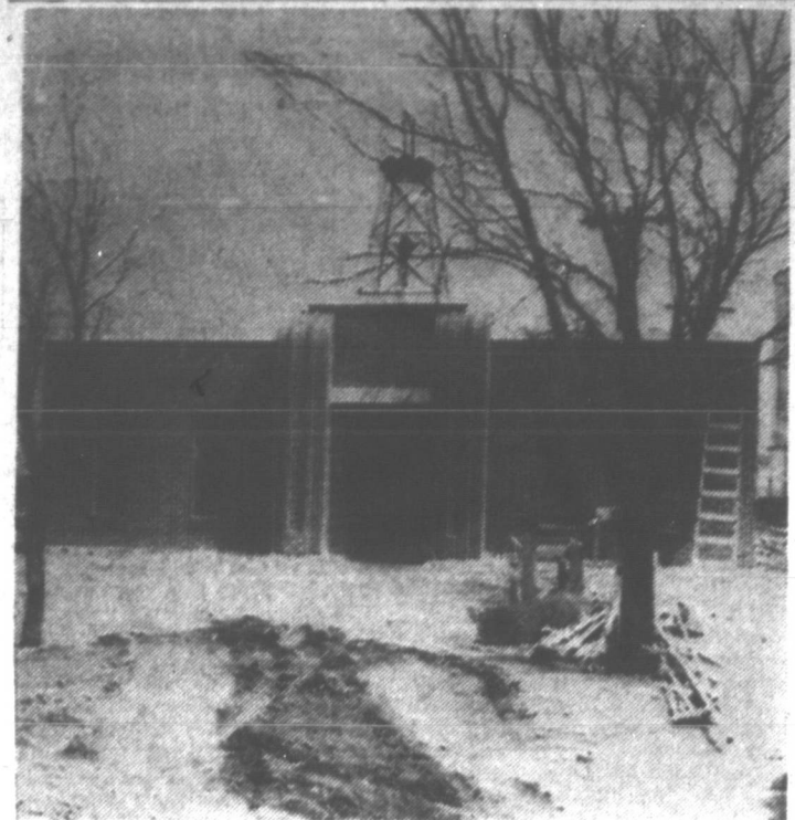
NEW PUMP STATION ANNEX—Water department's new annex to the S. Hobart pump station was built to house two huge pumps in the department's expansion project. (News Photo and Engraving)
