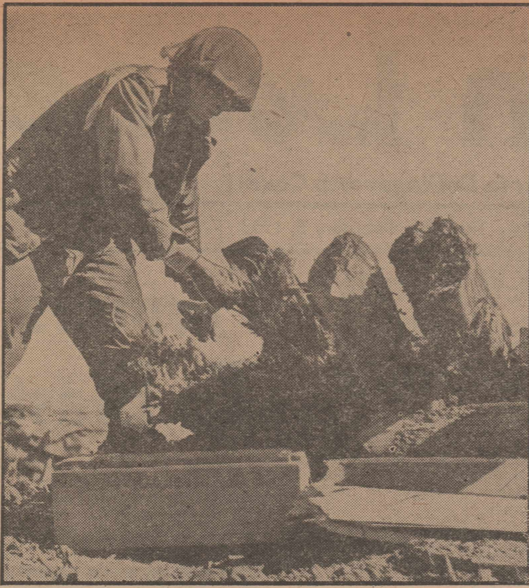
BUNKER FIXIN' ON OLD BALDY —Pvt. John Micheletti of Providence, R. I., takes time out from fighting in Korea to repair his bomb-busted bunker atop Old Baldy, which was banged up during the night by the enemy. Battle-scarred Baldy, now practically a barren peak, has been fought over viciously by both sides.
