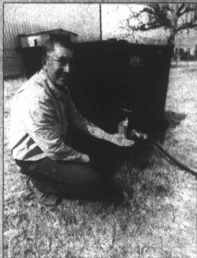
THE FUTURE OF WATER — Joe Rivera has an Atmospheric Water Generator in Colorado City. It's a new technology that converts humidity in the air into fresh water, and he's hoping it could be the start of something good for his hometown.
