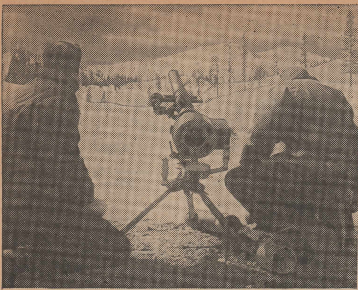
TARGET: 1960 — Zeroed in on the "White Death" — a potential avalanche—are U.S. Forest Service avalanche expert Montgomery Atwater, left, and John Mortiz, chief of the Squaw Valley, Calif., ski patrol. Concussion of shots from the 75-mm. recoilless rifle is designed to shake loose any mass of snow that threatens to become a death-bearing avalanche. Conclusion reached from results of the test: Squaw Valley can be made reasonably safe for holding of the 1960 Winter Olympics.
