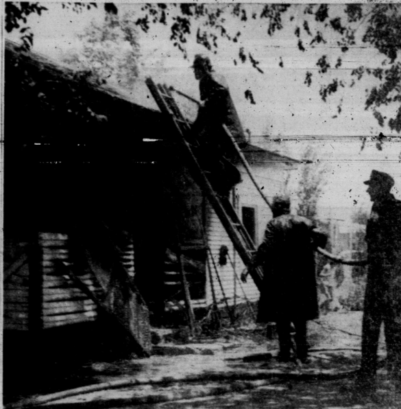
ATTACK FROM ABOVE —Firemen scaled the walls to fight the blaze that swept through Mrs. Isom Evans' home at 424 Twenty-eighth Street Tuesday afternoon, destroying the attic, back porch, kitchen and one bedroom and heavily damaging the front of the house. Above, firemen mount the roof to extinguish the fire still raging in the attic after they had controlled that in the lower part of the house. The fire originated on the porch.
