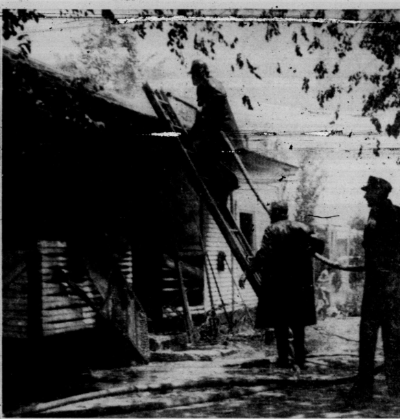
ATTACK FROM ABOVE—Firemen scaled the walls to fight the blaze that swept through Mrs. Isom Evans' home at 424 Twenty-eighth Street Tuesday afternoon, destroying the attic, back porch, kitchen and one bedroom and heavily damaging the front of the house. Above, firemen mount the roof to extinguish the fire still raging in the attic after they had controlled that in the lower part of the house. The fire originated on the porch.
