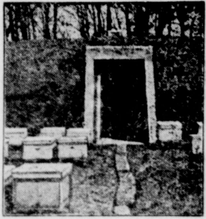
Concrete Bee Cellar.
