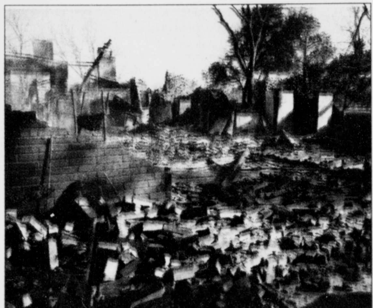
FLAMES REDUCED A once-beautiful home into a pile of rubble during Sunday's fire that consumed 9 occupied homes north of Colorado city, including that of Jerry Strain. Photo courtesy David Redwine
