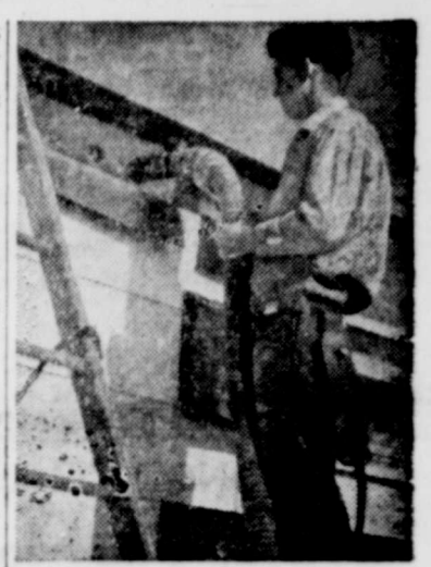
Mineral wool is being blown into walls of this house to form a tight blanket that will keep heat in, prevent drafts, and cut fuel bills, year after year.
