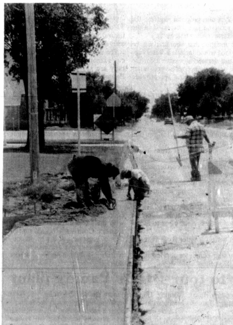
Workers smooth out a concrete valley between Murphy and Barnes Streets as part of the city's street renovation program Tuesday afternoon. From left are Dan Fletcher, John Jimenez and Richard Preciado of Wood's Concrete out of Amarillo.
