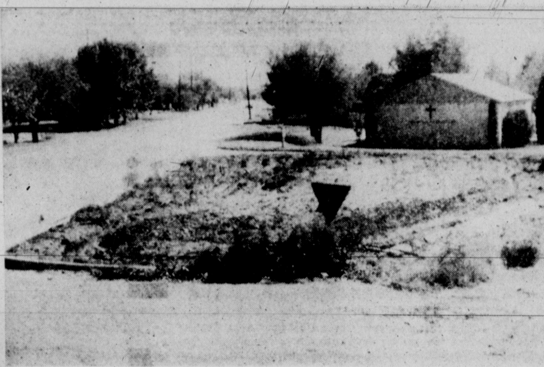
Project Beautification Site
