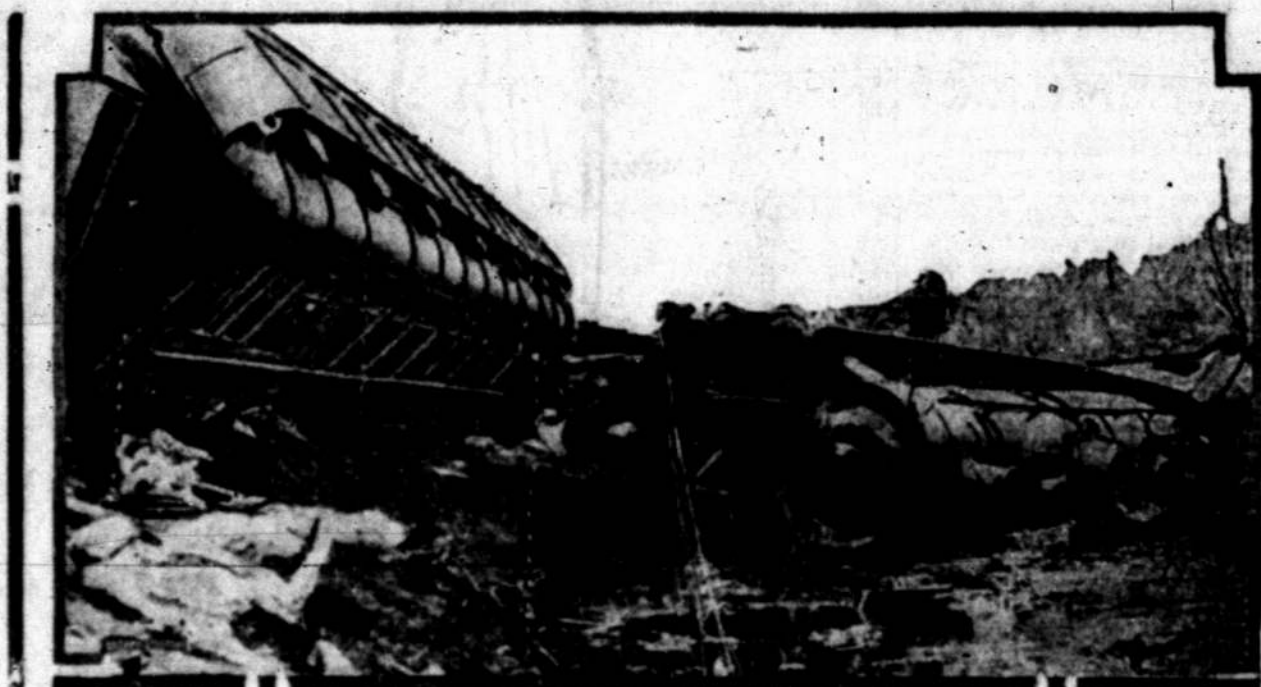
Three trainmen were killed and two others badly injured and many passengers cut and bruised when the explosion of an engine boiler wrecked the crack train, "Cape Codder," the New Haven summer express, on its initial trip, at Kingston, R. I. This view of the wreck shows two of the overturned cars, and the locomotive half buried in a swamp.
