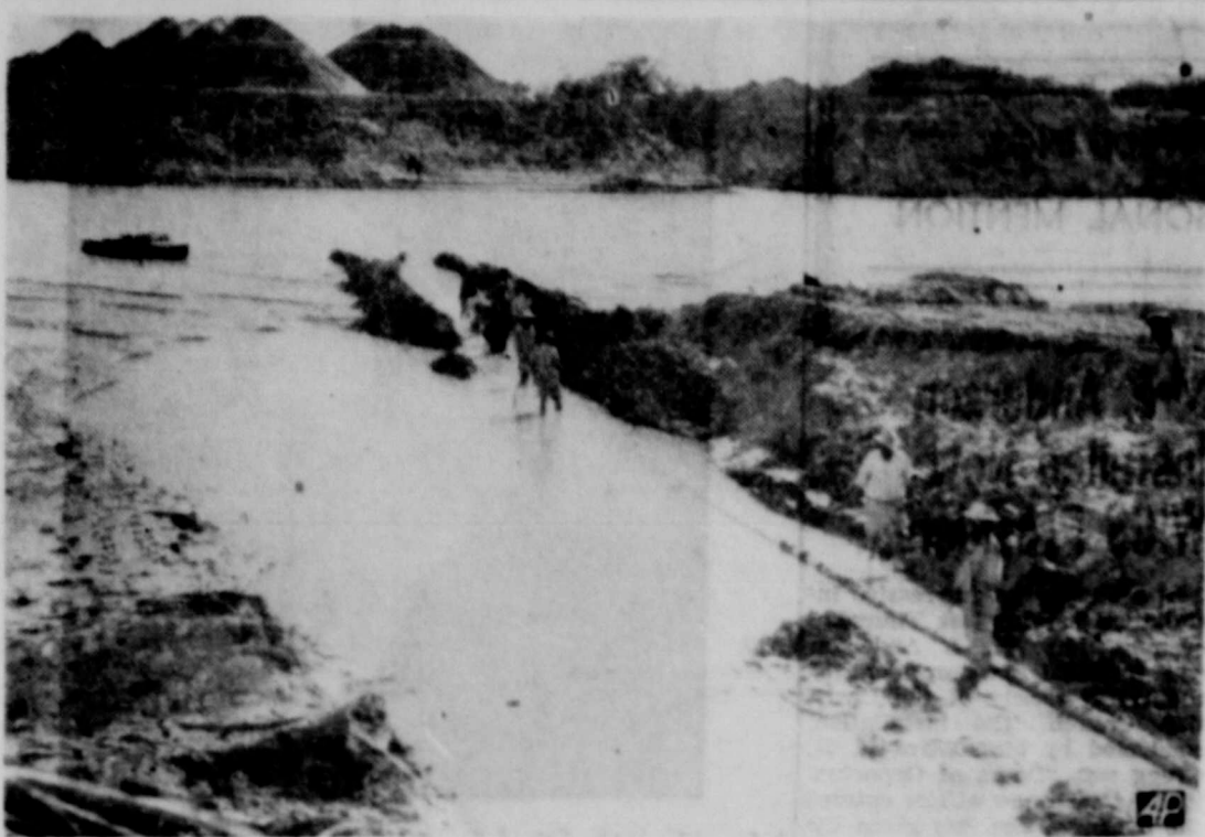
GAS LINE TO MEXICO —Workmen are shown installing a section of pipe in a trench cut across the Rio Grande a mile east of the International Bridge at Hidalgo, Tex. The $4,000,000 line, when completed, will be 151 miles long and will carry natural gas from the South Weslaco field in Hidalgo county, near the town of Weslaco, Tex., to industrial plants in Monterrey, Mexico. The Mexican shore (Retnosa) is in the background.
