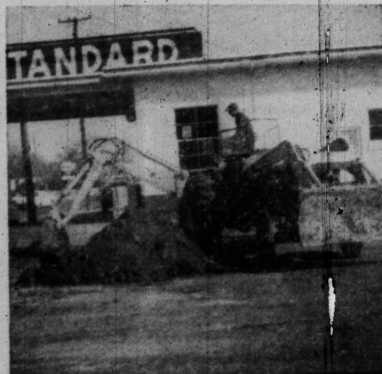
A NEW BACKHOE purchased this year is shown in operation. A water department employee is shown making a hole to repair a water leak.
