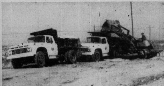
CITY CREWS haul many tons of material each year to maintain dirt streets in the more sparsely developed areas of the city.
