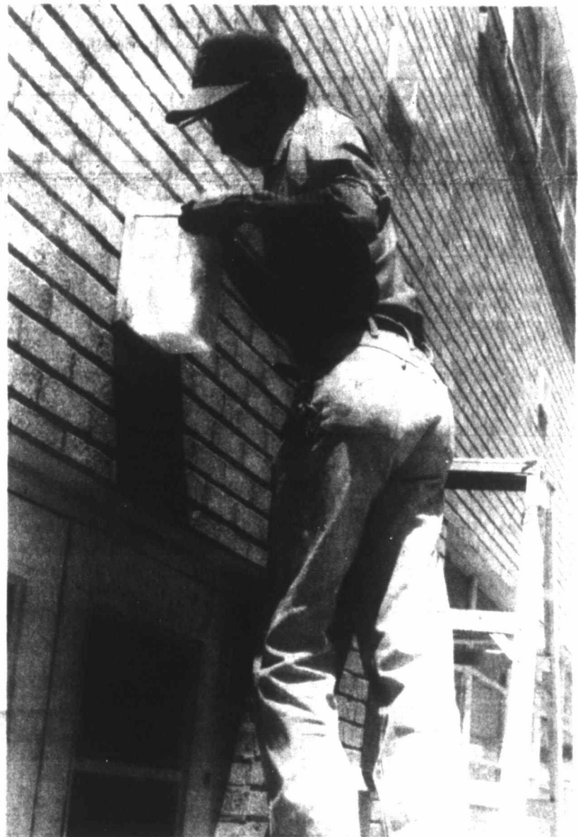
BACK TO SCHOOL: Rene Garcia makes some last minute repairs at Colorado Middle School in preparations for the new school year. This is the annual back to school issue. Supply lists for the local schools, school calendars and names of the local teachers are listed in this years edition.
