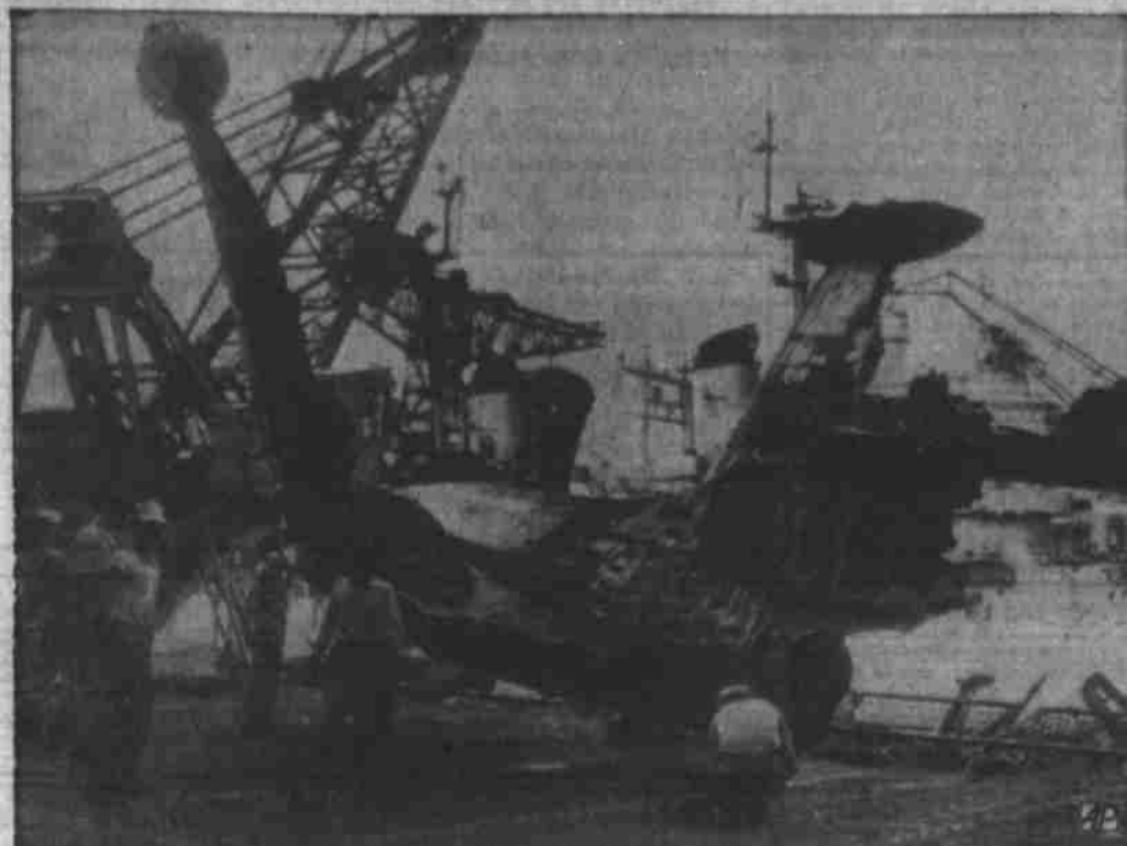
Damaged Plane Taken From Boxer
