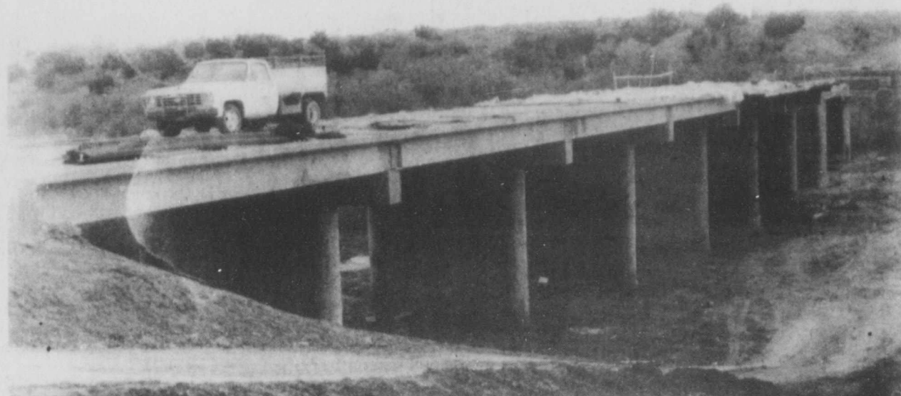
CONSTRUCTION ON A BRIDGE on the south Service Road of Interstate 20 is progressing very well. County Commissioner Johnny Shackelford said that the bridge would allow drivers to get from Westbrook to Colorado City without getting on the Interstate.
