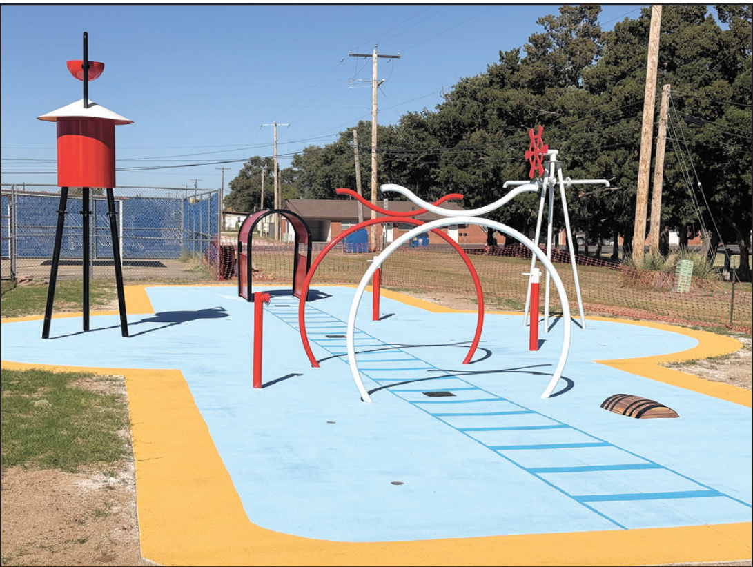
Just add water — Work on the new splash pad at the Friona Swimming Pool is nearing completion. The project should be wrapped up sometime in November.
