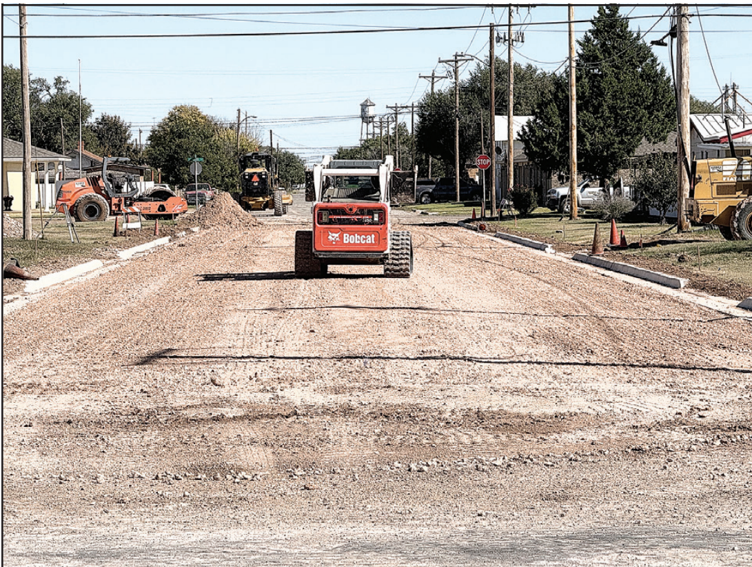
Takin' It To The Streets — Bermea Construction is currently building the newest paved street in Friona. The Curbing/Paving Project on 7th street between Grand and Ashland is well underway.
