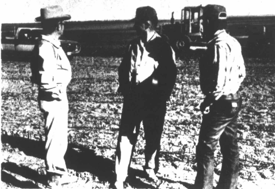
TERRACE CONSTRUCTION IS UNDERWAY on the D.M. Smith farm in the Rodgers Community. Costshare assistance was received through the ACP Program. Observing (left to right) are J.T. Rich, D.M. Smith and Van Mills.
