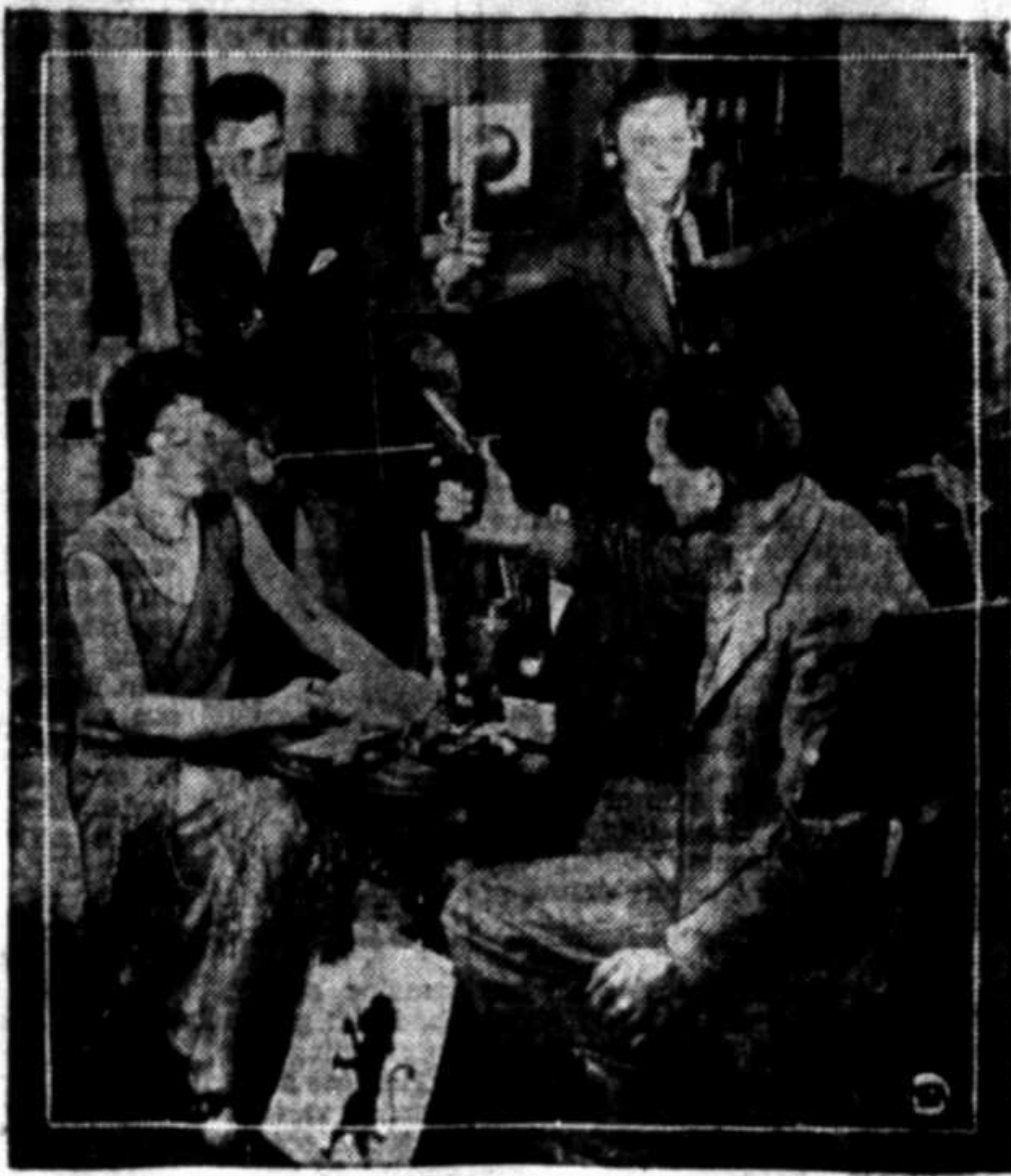
The cameras here contain the electric eyes, reproducing by television a play enacted in the studios of WGY at Schenectady, N. Y.
