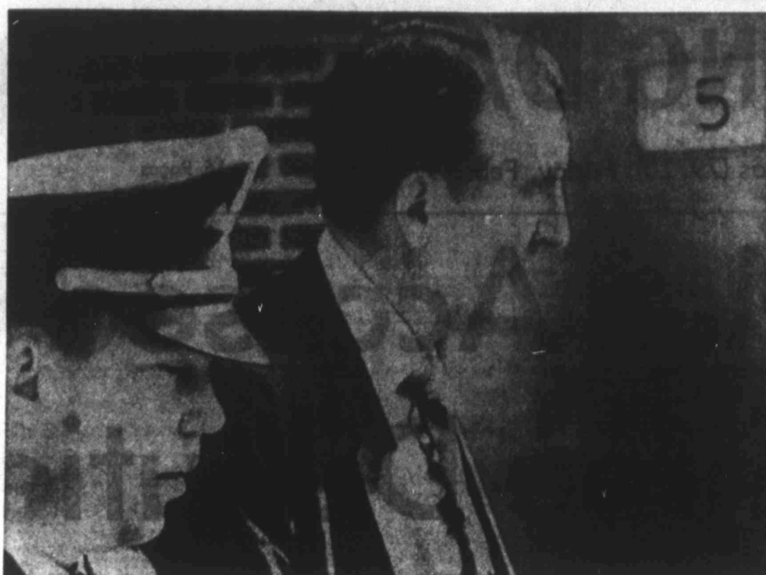
CALLEY AND KAY ARRIVE At Building Five For Trial
