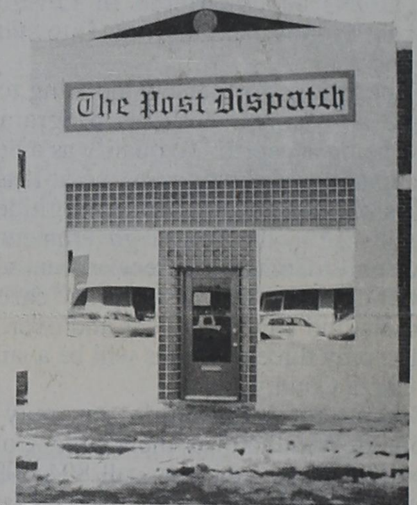
The Post Dispatch renovation was completed under the Main Street Project approved design and low interest loan program.
