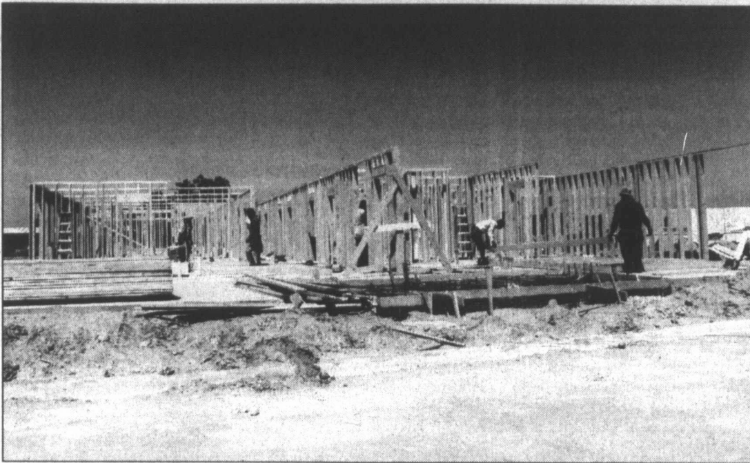
GOING UP FAST – Framing work has begun on the Studio 6 motel being constructed west of the sports complex. Adam Keller from M&L Builders said that he hopes to have the motel finished before the end of the year.
