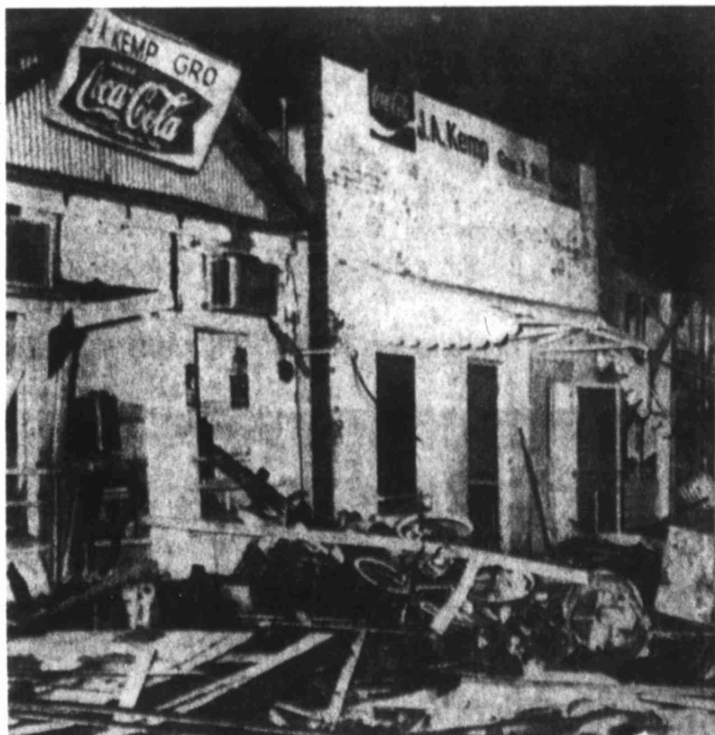
DOWNTOWN INVERNESS — Debris is piled high in the street in downtown Inverness, Miss., that was hit hard by a tornado.
