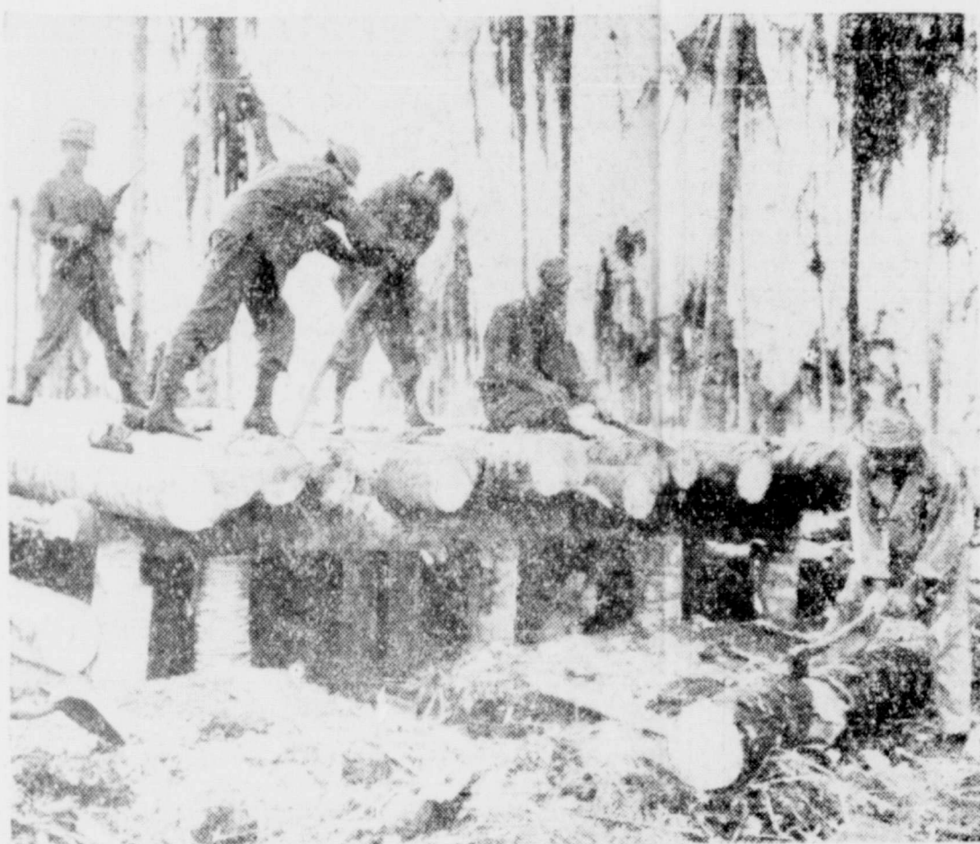
WARTIME LOG CABIN—Constructing a command post near Arawa, New Britain, infantrymen use heavy logs to protect vital equipment from mortar, light artillery shells and light aerial bombs. Photo shows soldiers completing roof of the shelter.
